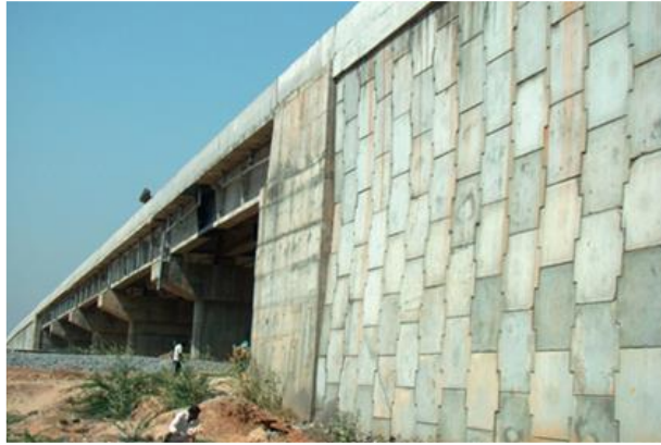
Figure 10.3. Photograph of the RE wall in Hyderabad-Bangalore highway in Anantapur [25]
