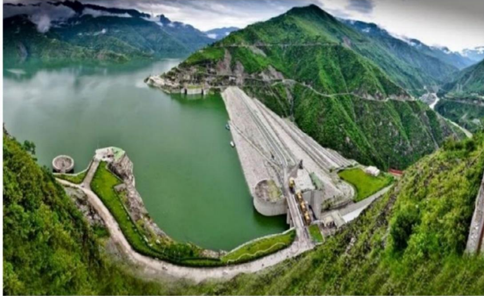
Fig 7.2.1. Tehri dam (India). The dam is one of the highest rockfill dams in the world and is located in seismic zone-V (Bureau of Indian Standard, 2016). Located on river Bhagirathi, the dam is a part of pumped storage scheme with Tehri being the main dam on upstream, and Koteswar dam (gravity dam) about 22 km downstream (Jazayeri & Moeini, 2020).
