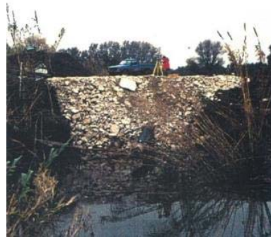
Figure 4.14 Scenario n°6: Contact erosion between gravel and silt (case of breaches repaired in emergency situations with permeable materials).
