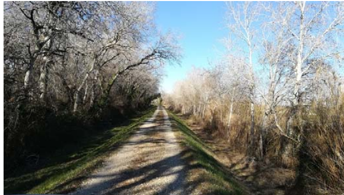
Figure 4.11 Scenario 3: Breach by concentrated leak erosion in a root of dead tree.
