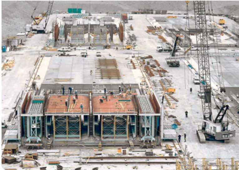
Figure 4: Close up of IMT structure being constructed at Port Kembla (courtesy of Ms Margaret Rush)
