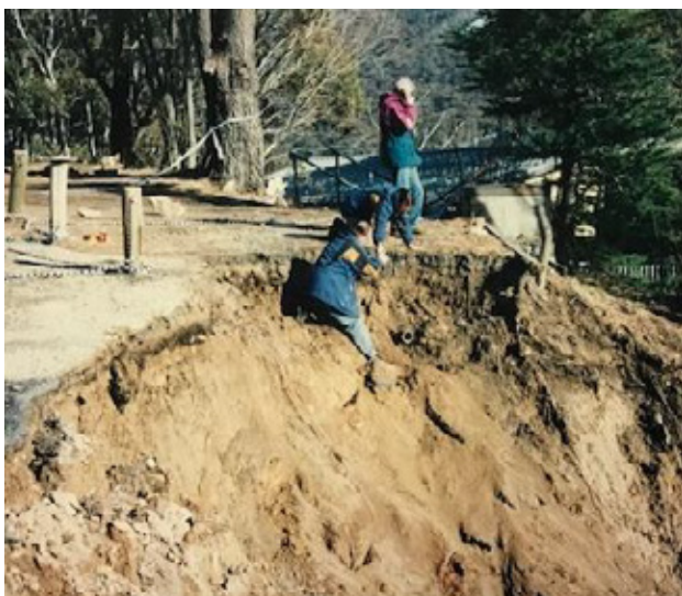
Figure 2: Broken AC pipe in landslide scarp
