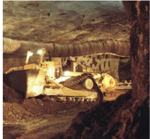
Photograph 2: D10 bulldozer used for bulk excavation in the cavern
