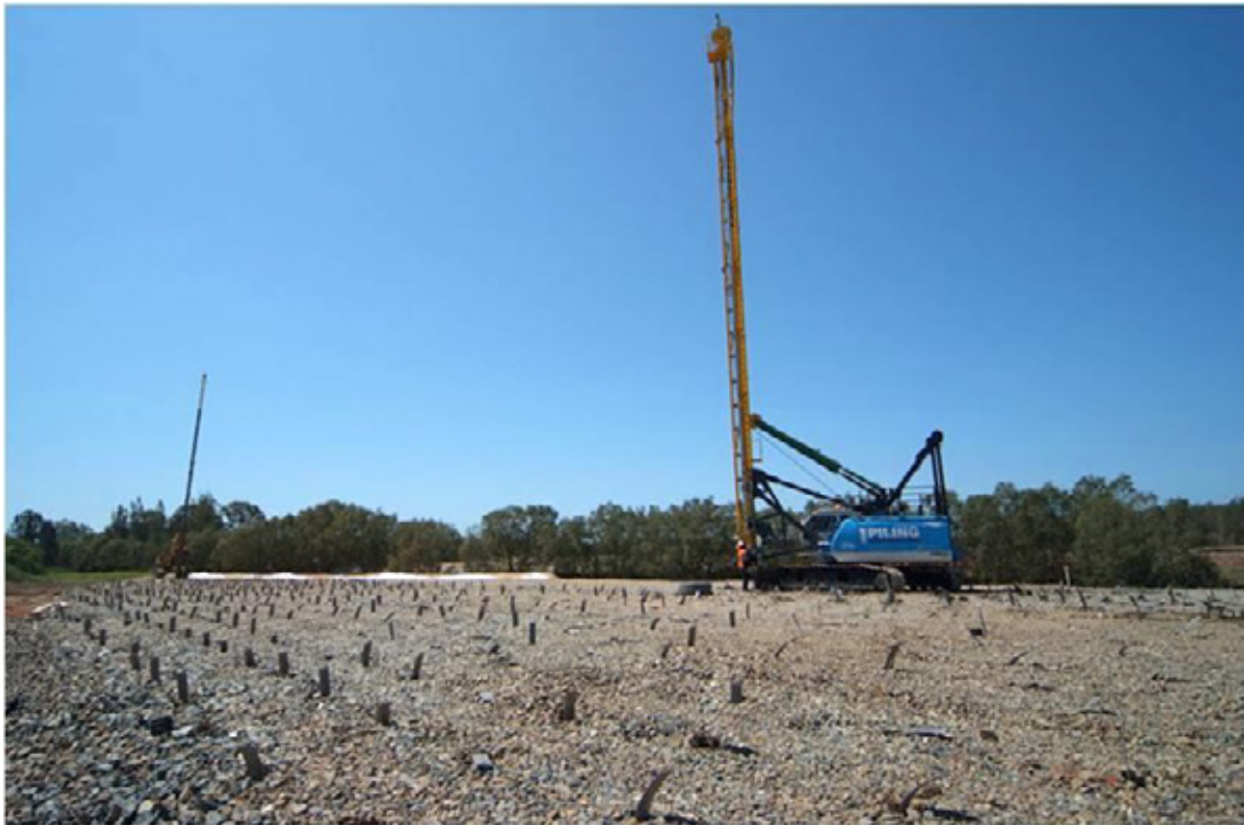
Figure 4: Wick drain installation
