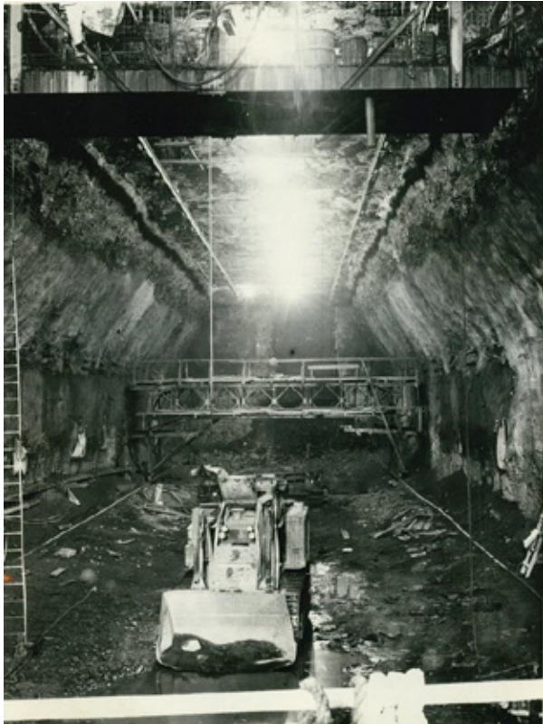
Figure 1: Poatina underground power station during excavation
