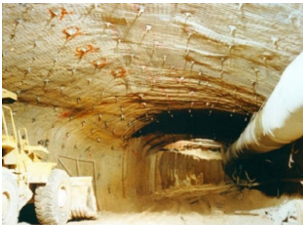
Photograph 1: Excavated vehicle access tunnel connecting to cavern in the distance
