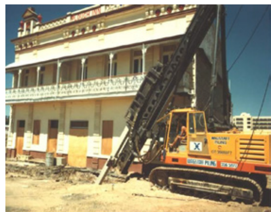
Expo '88 anchor piles
