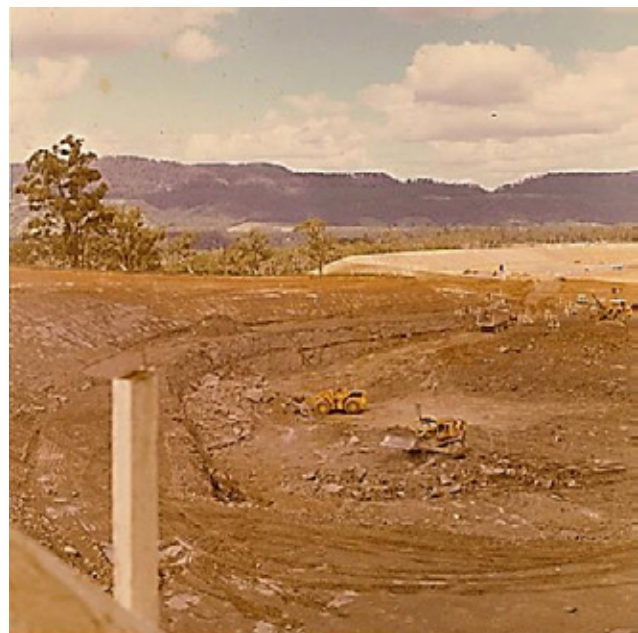
Figure 7: Kangaroo Valley Power Station Excavation following the 'Big Bang'
