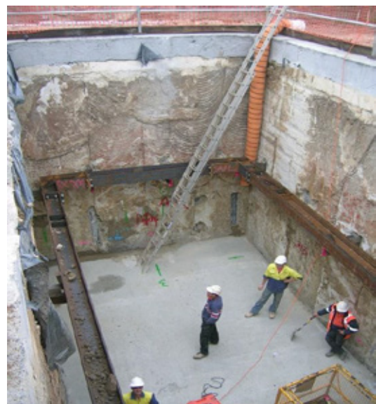
Soil mixing CSM method
