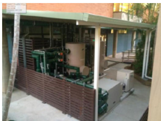
Figure 8: Above ground components of Gatton test
