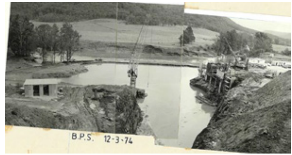
Figure 4: Bendeela Power Station flooded
