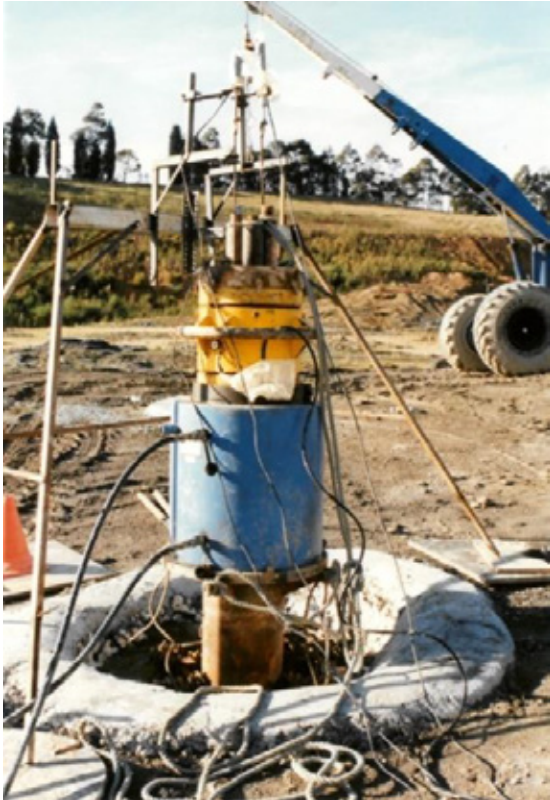
Figure 7: Static load test of socketed pile at Scoresby test site
