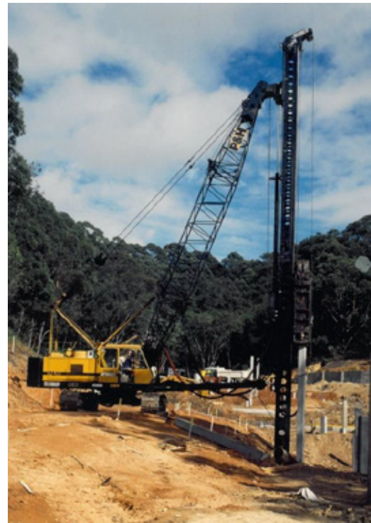
Earlier innovations – hydraulic pile rig /hammer
