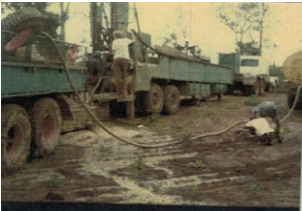
Drilling- open hole - mud stabilisation- downhole logging, Mae Moh, Thailand 1979
