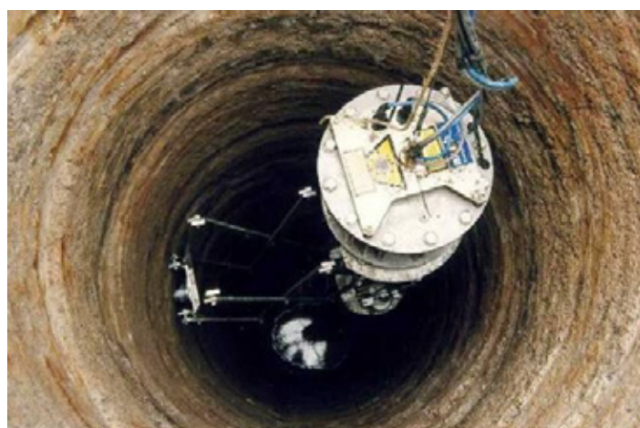
Figure 6: Down hole socket side roughness profiling device
