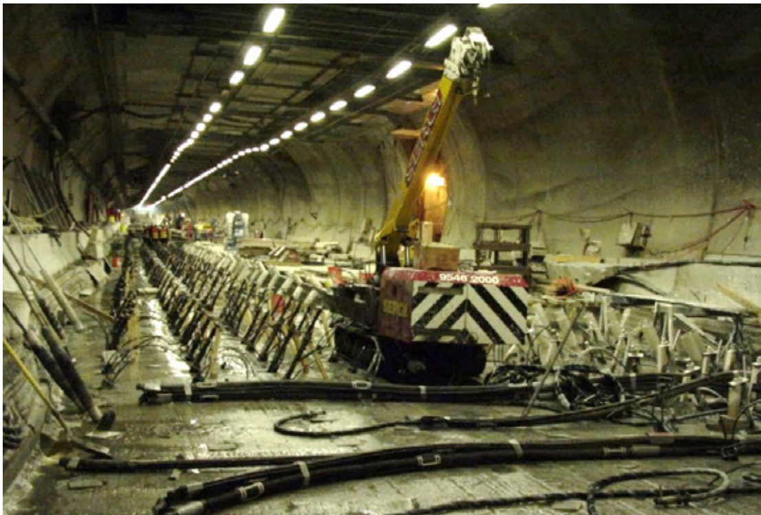
Photograph 1: Multi-anchoring of failed slabs
