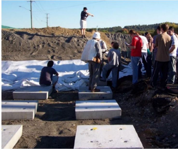
Arthur Love explaining the principle of a piled embankment to engineering students from the University of Newcastle at Five Islands in 2005
