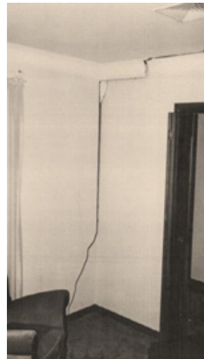
Fig. 4: Corner crack
