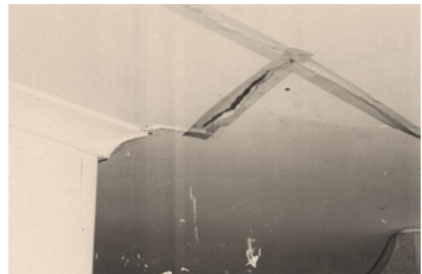
Figure 11: Ceiling crack
