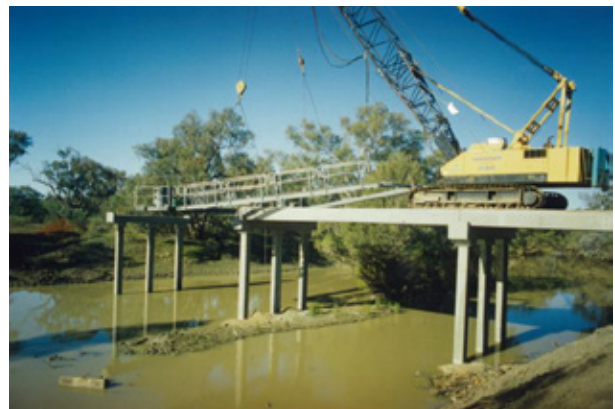
Installation of M-lock bridges
