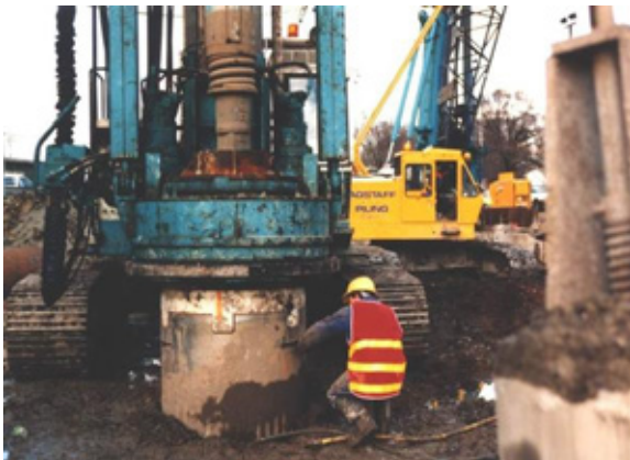
Secant piles – cased – hard/hard
