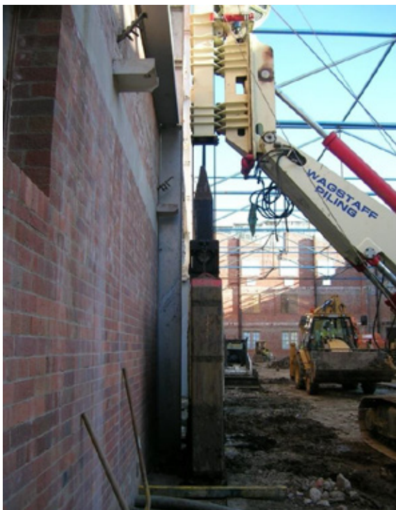
Diaphragm walls – small and thin
