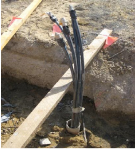
Figure 4: Double loop prior to grouting at EBSS
