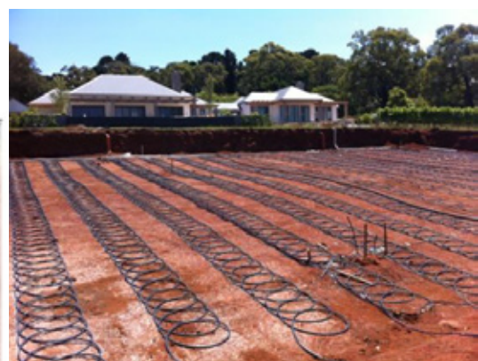
Figure 2: Horizontal loop system at Main Ridge before backfilling
