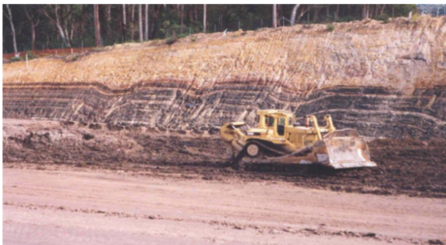
Effects of mine subsidence in an underlying seam, evident in an overlying seam exposed during construction of the West Charlestown Bypass in 2000
