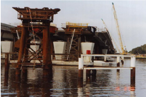
Narrows Bridge construction
