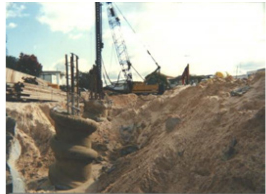
Purpose built rig – Campile
