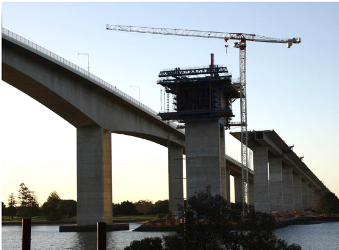
Figure 6: Construction of the New Gateway Bridge
