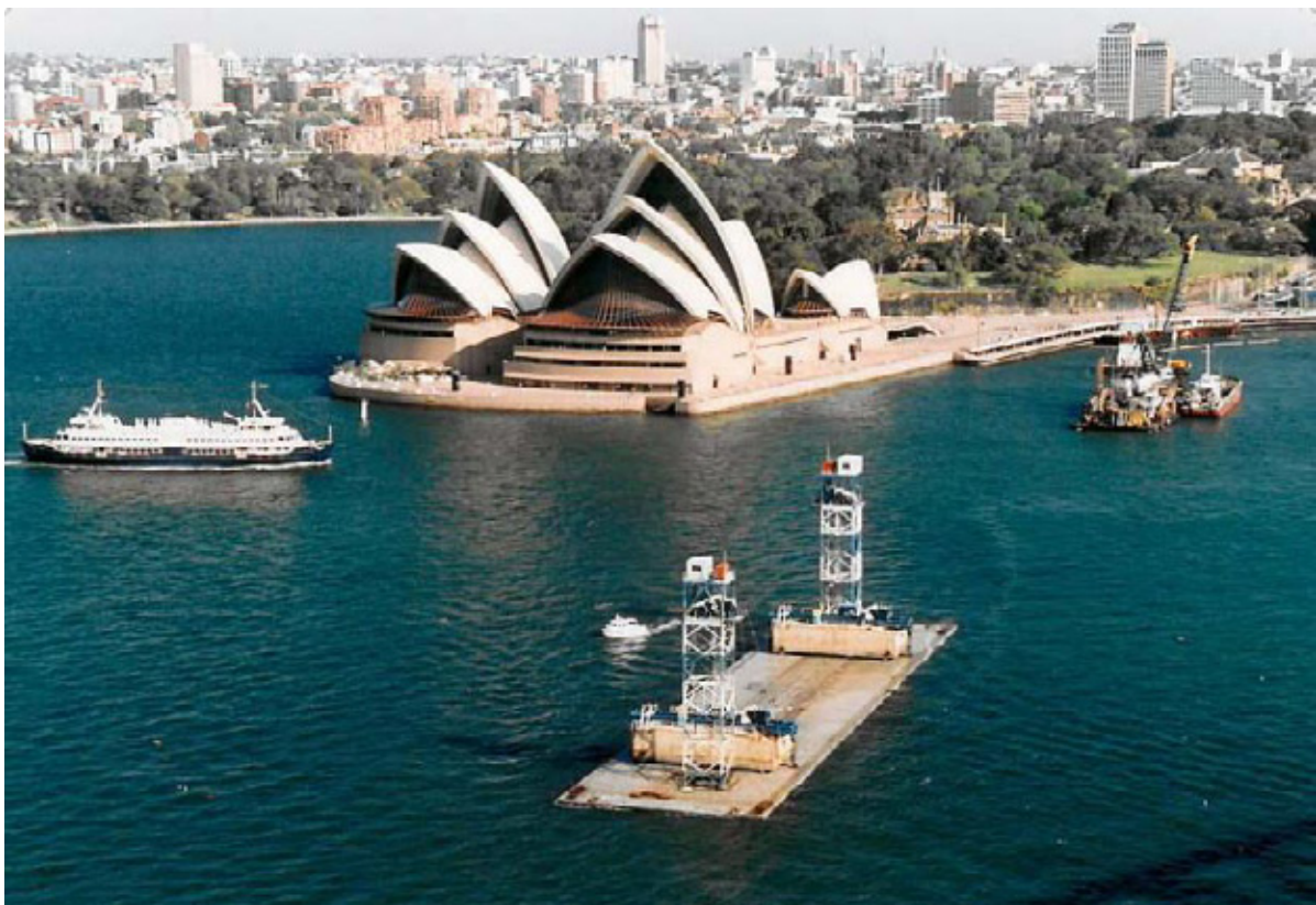
Figure 6: An IMT unit in position ready for sinking (courtesy of Ms Margaret Rush)
