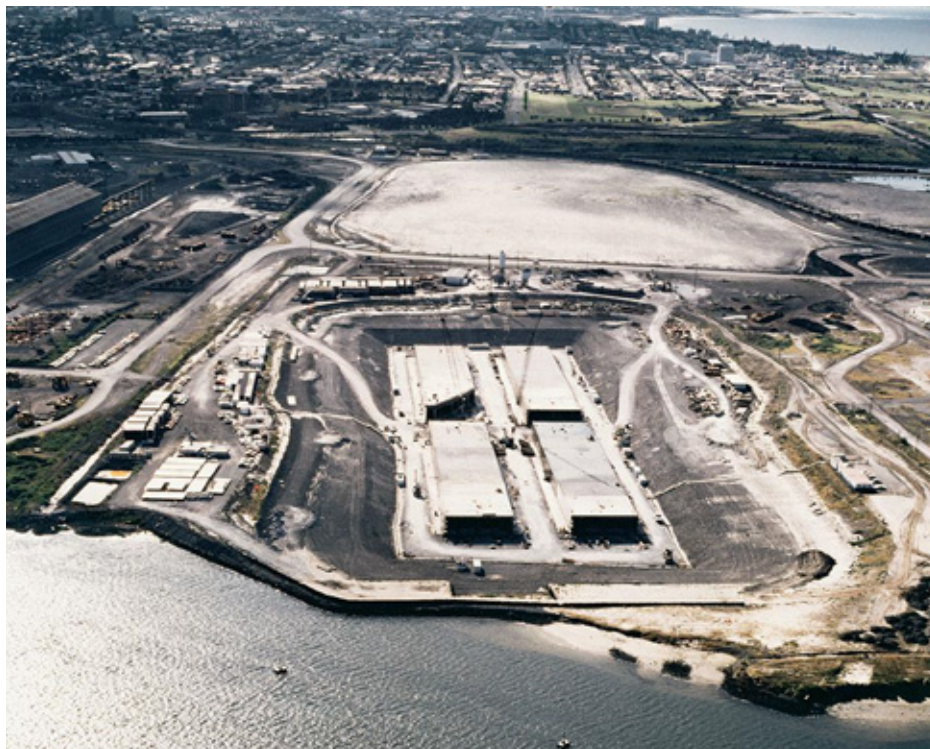
Figure 3: Casting Basin for the Construction of the IMT Units at Port Kembla (courtesy of Transfield)
