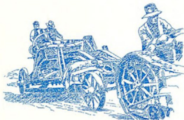
ROAD CONSTRUCTION GRADING EQUIPMENT OF THE 1930'S NOWADAYS HIGHLY AUTOMATED AUTOGRADE MACHINES ARE USED FOR SPREADING AND SHAPING
