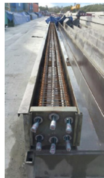
Figure 9: Energy pile for Brisbane River sediments
