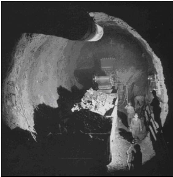
Figure 5: Eucumbene-Tumut tunnel during excavation (Endersbee, 1999)
