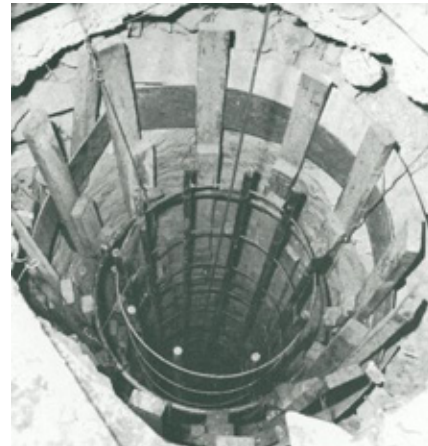
Down the dyke with timbers & shafts set
