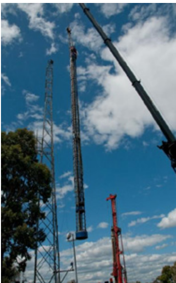
Figure 7: Instrumented energy pile cage for Monash test facility
