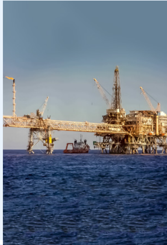
North Rankin A Platform Photograph courtesy Harry Poulos
