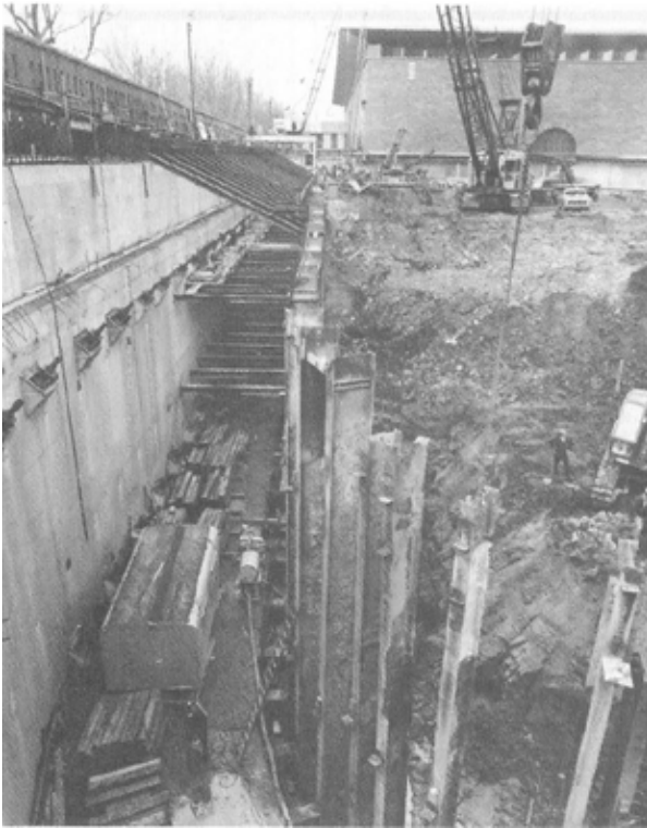
Plate 2: Trench construction along St Kilda Road
