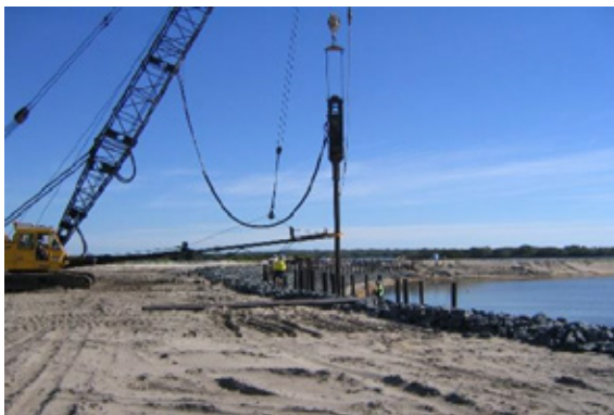
Purpose built rigs- long reach
