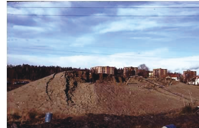
Fig. 4. Photograph after failure
