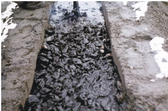
Fig. 2. Injecting hot bitumen into gravel matrix
