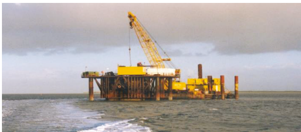
Fig. 1. Tie-in Chamber during construction
