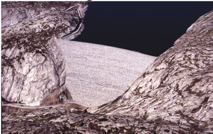
Fig.1. Photograph of Svartevann dam
