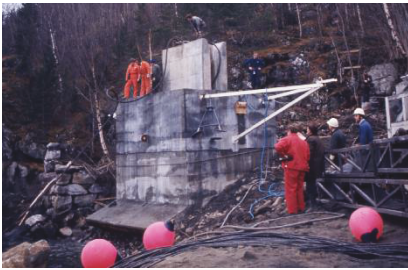
Fig. 1. Anchor block on launch skid prior to deployment
