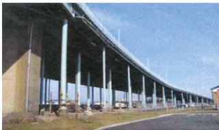
Fig.1. View of part of the bridge
