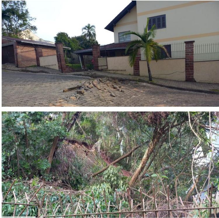
Figure 4. Cracks in streets and instability suggesting large scale ground failure.
