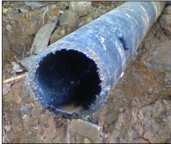
Figure 2.23 Outlet of a subsurface drain installed at the site
