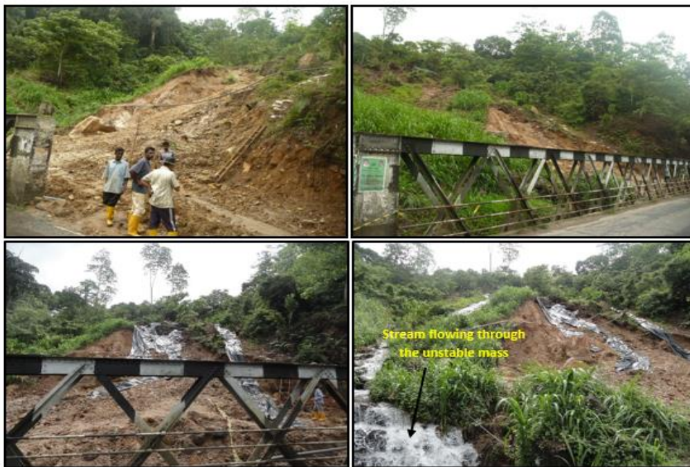
Figure 3.2 : Landslide occurs on 22 nd June 2014 (National Building Research Organisation, 2014)
