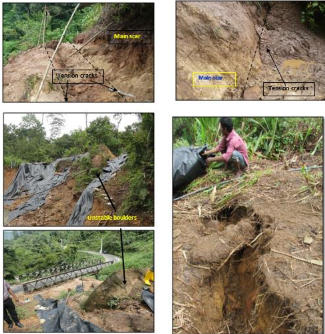
Figure 3.4 : Tension cracks and unstable boulders (National Building Research Organisation, 2014)
