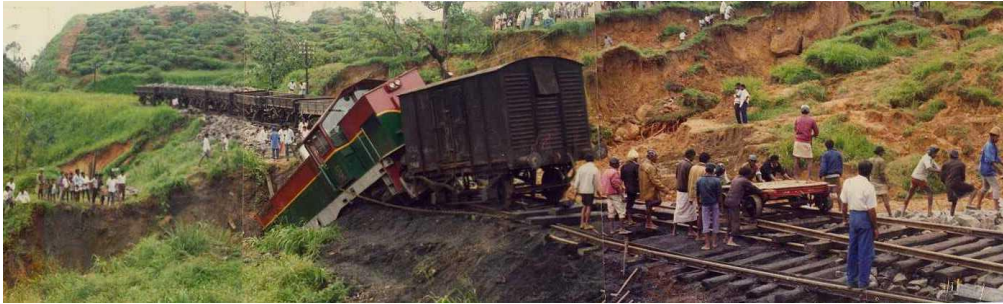
Figure 2.25 : Watawala Landslide after Failure (Rajaratnam & Bhandari, 1994)
