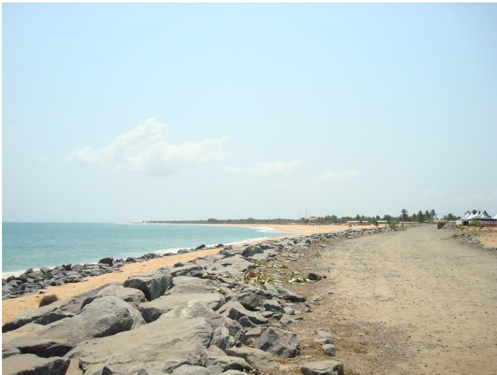
Maritime dyke protection
